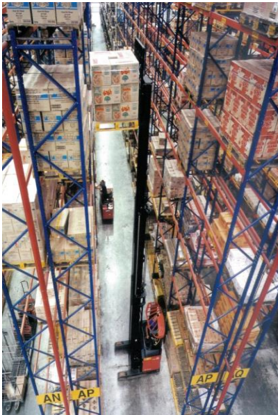
Indoor, free standing, 12.5 m, reach truck operated
